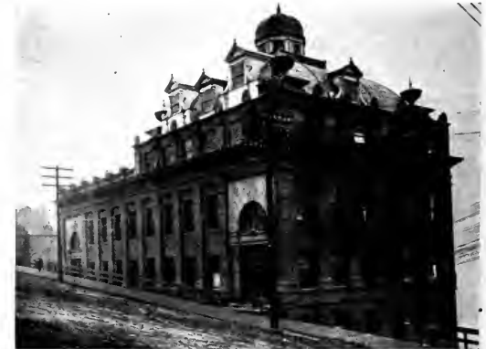
FIG. 9.—SEATTLE SUB-STATION AND OFFICE BUILDING.
